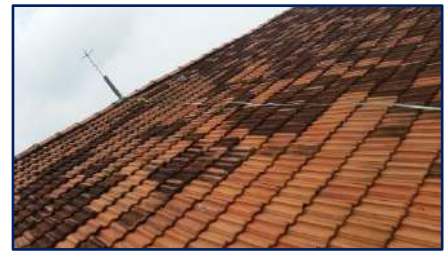
Roof - Main Building
