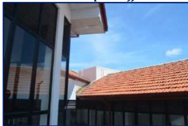
Overhead Water Tank
